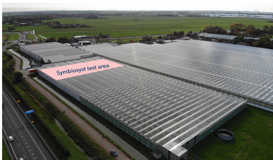
Figure 29: Existing greenhouse and display of the SYMBIOSYST test area
