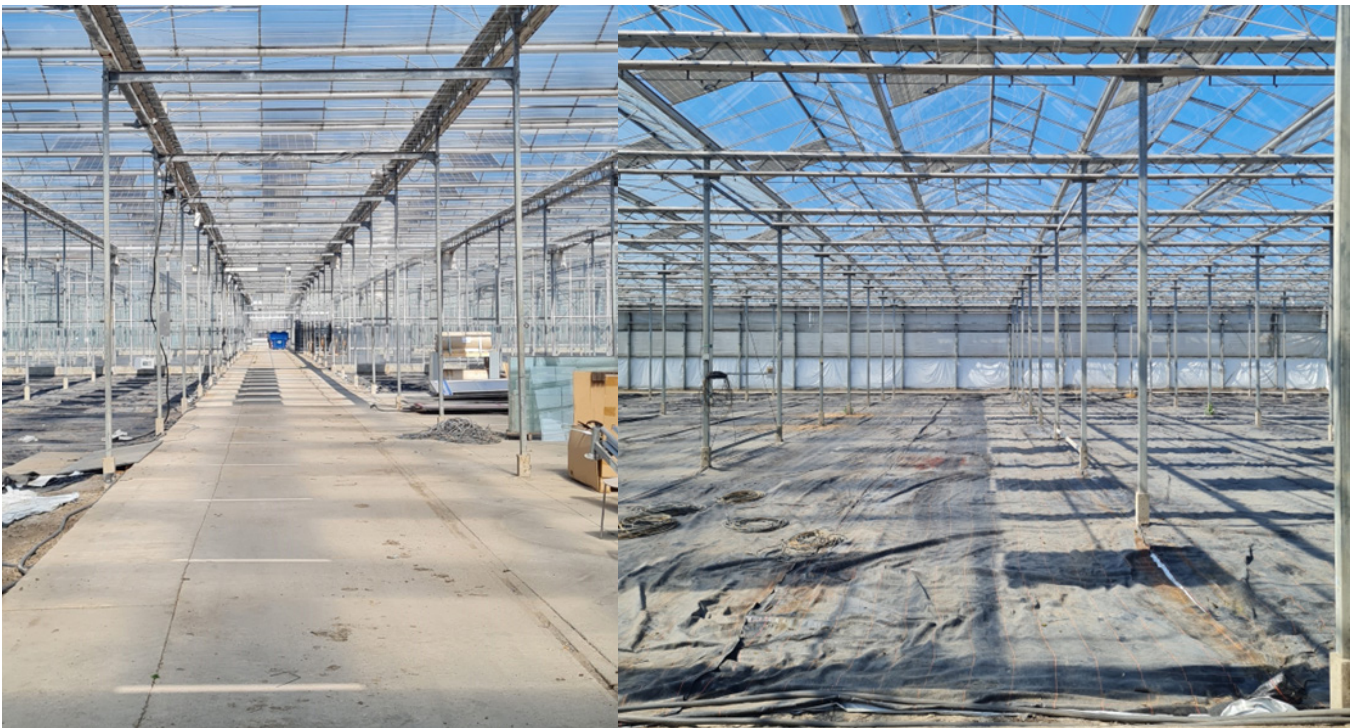
Figure 43: The effect of diffusive PAR+ coating with PV-panels on top of the greenhouse. The shadows appear to be less hard due to the 35% hortiscatter.
